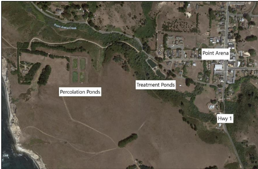
Figure 3-5: Point Arena WWTP Facilities
