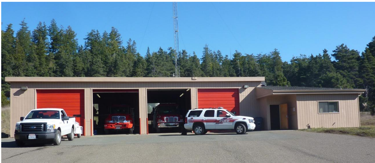
Main Fire Station 39215 Baptist Church Street Gualala
