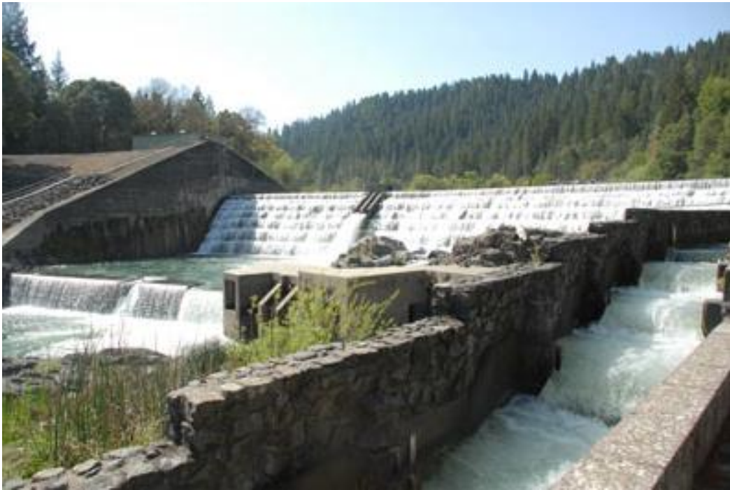
Figure 3-2: Cape Horn Dam and the Fish Ladder at the Potter Valley Project Source:(PVID, 2024)
