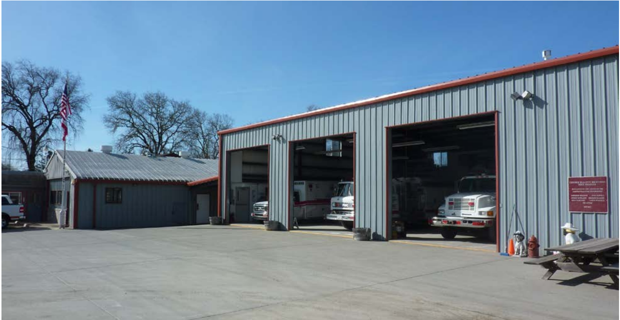
Main Station - George Elliott Memorial Fire Station
