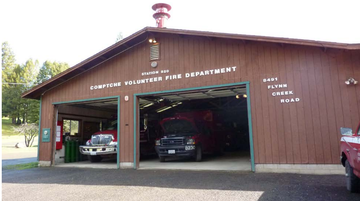
Main Fire Station Station 820 8491 Flynn Creek Road Comptche Comptche Community Services District
