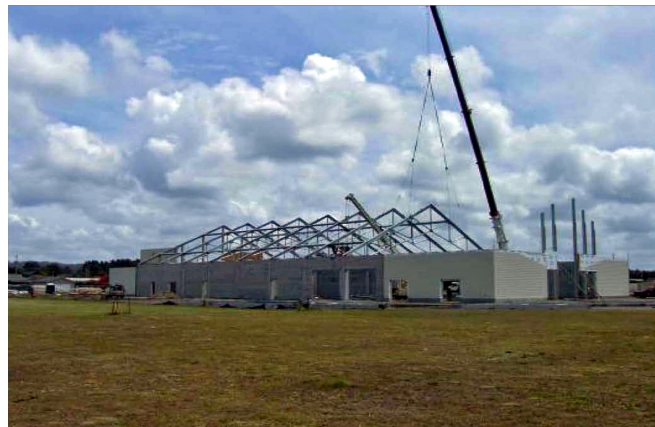
Image 3 - - Natatorium Construction Summer 2007
