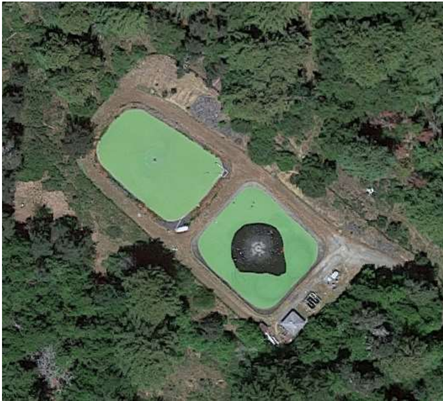
Figure 3-3: Arial View of Wastewater Treatment Plant
